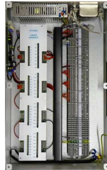
Qube RIO – Remote IO Mounted on Lift Cabin
